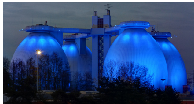
Thermal pre-treatment of waste activated sludge before anaerobic digestion can increase the biogas output and is one of the processes studied in the "IntenKS" project
